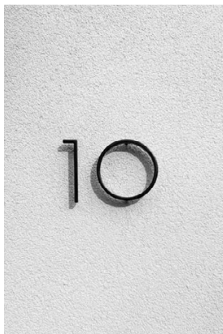
TENANCY SIGNAGE FIXED METAL LETTERING
