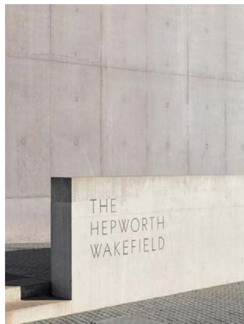
DEVELOPMENT SIGNAGE DEBOSSSED LETTERING IN CONCRETE
